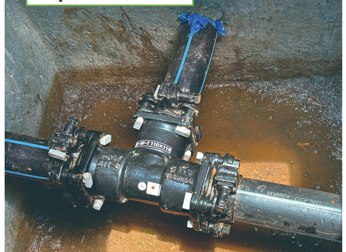
Equal Tee Installed
