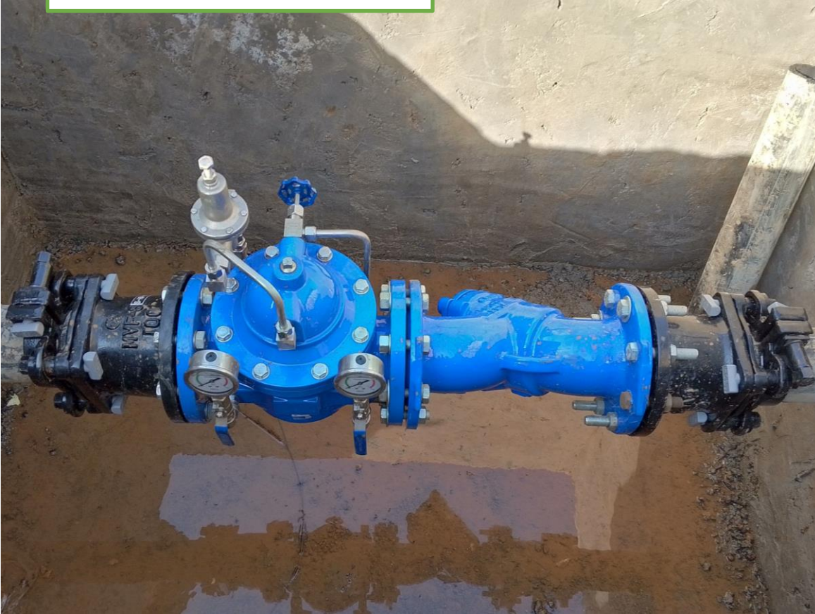
PRV Installation
