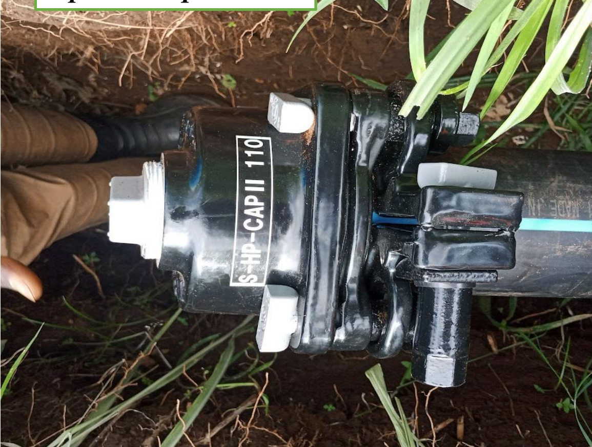
Pipe End Cap Installed
