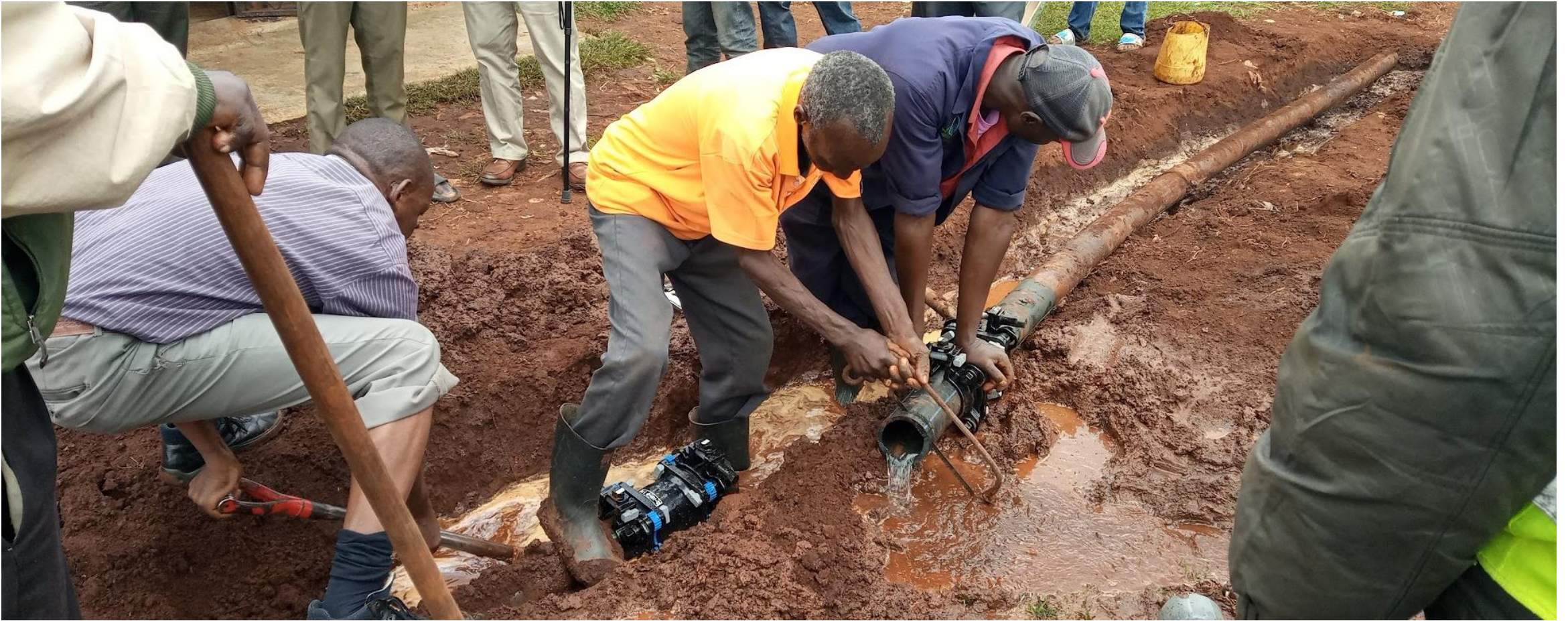
Repairing HDPE pipeline in Kericho Kenya
